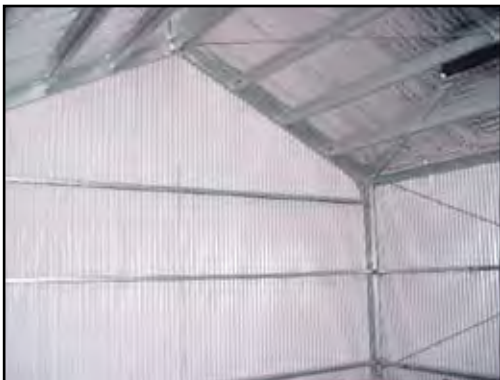
Before Spray Foam Application
