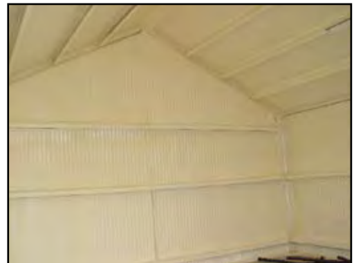
After Spray Foam Application
