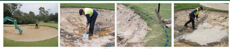
Remove sand from bunker; cut, shape and smooth bunker as desired. Spread 10mm of fresh sand into the bunker without covering the drains.
