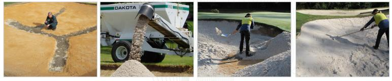
Once the **Klingstone**® is cured apply and spread fresh sand to bunker and it's ready for service.
