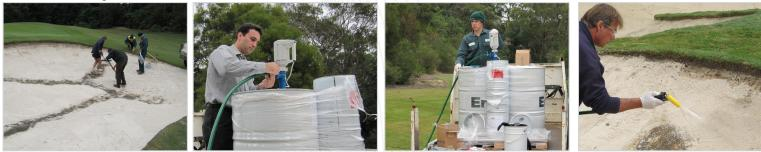
Spray apply Klingstone® to fresh sand. **Klingstone**® is a single component polyurethane applied with a simple water pump, garden hose and spray nozzle.
