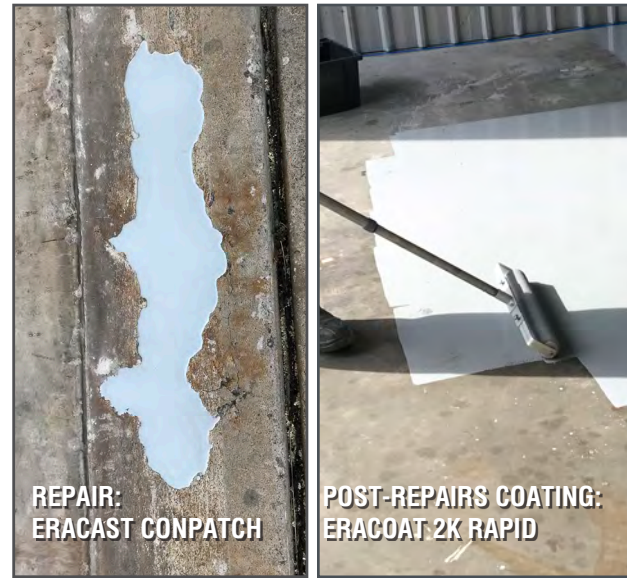
Concrete floor - Repaired with Eracast Conpatch
